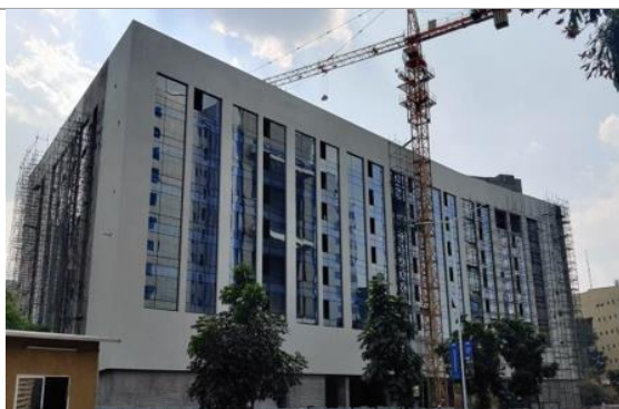
B-22 (Hotel): Structure Completed
