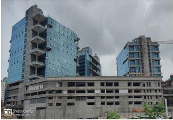
Building 5 – Podium level RCC work in progress
